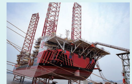
JWFC SUNRISE under construction in Shanghai
