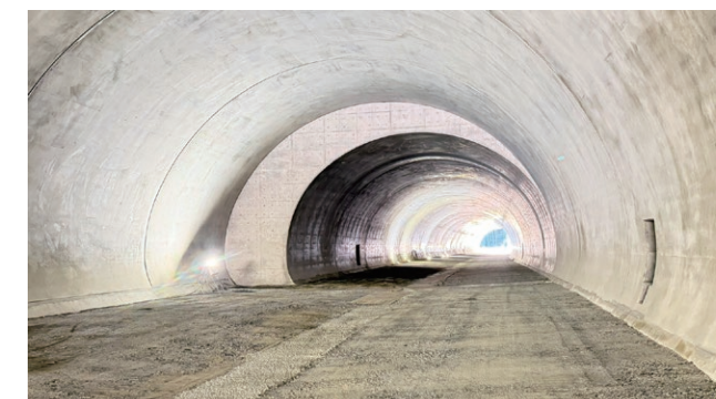
Susami-Kushimoto Road Esumi No. 1 Tunnel construction Customer: Kinki Regional Development Bureau
