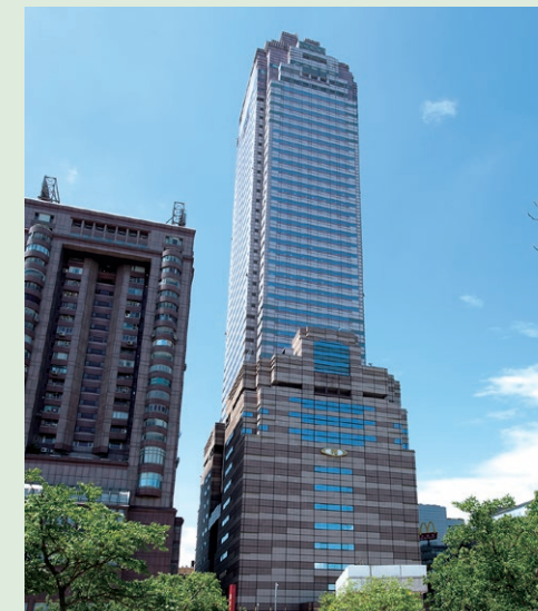
Super high-rise large-scale mixed-use commercial building Shin Kong Life Tower
