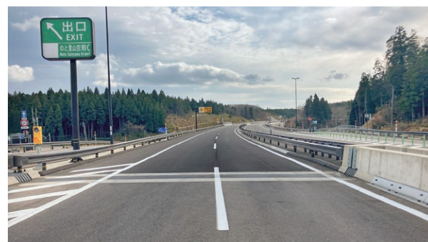
Noto-Satoyama Expressway, where early recovery was achieved using precast step slabs for repairs
