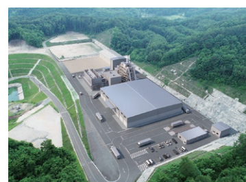
litate Mirai Power Plant
