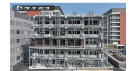
Innovation Airport (Ishikawa Prefecture) Customer: Kanazawa University
