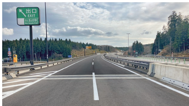
Noto-Satoyama Expressway, where early recovery was achieved using precast step slabs for repairs
