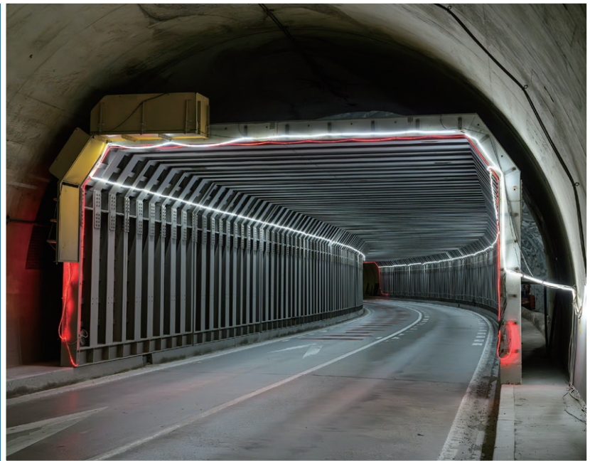
Steel protectors installed to reinforce the existing tunnel
