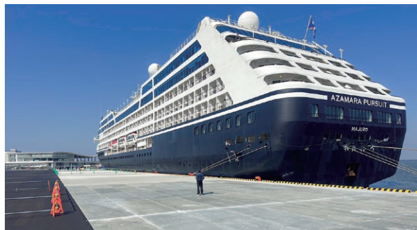
Kanazawa Port Cruise Terminal restored using PRC slabs
