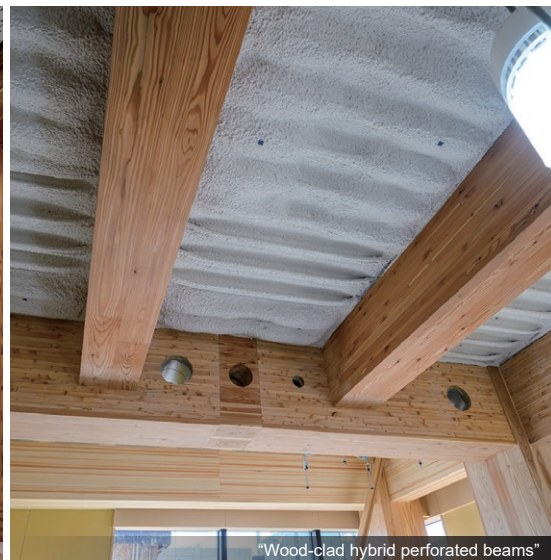
"Wood-clad hybrid perforated beams"
