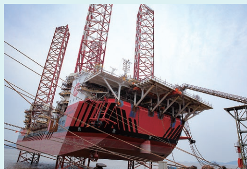
JWFC SUNRISE under construction in Shanghai
