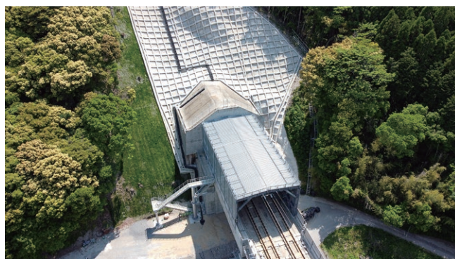
Kyushu Shinkansen (West Kyushu) track section between 17k5 and 44k2 Customer: Japan Railway Construction, Transport and Technology Agency, Kyushu Shinkansen Construction Bureau
