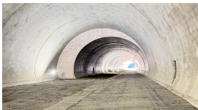
Susami-Kushima Road Esumi No. 1 Tunnel construction Customer: Kinki Regional Development Bureau
