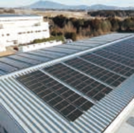
Experimental building (seam-jointed folded plate roof)
