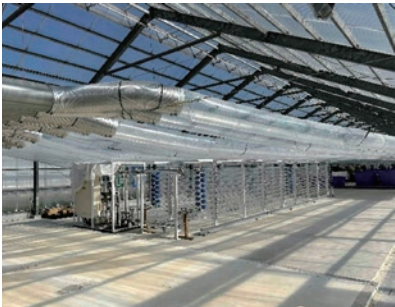
Algae Cultivation Equipment (photobioreactor)
