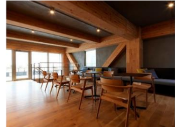
KININARU BLDG. Floors made of wood hybrid laminated wood (10F)
