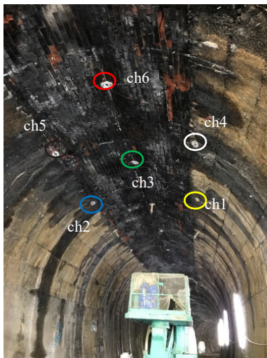
Photo.3 Monitoring points at the crown along the tunnel
